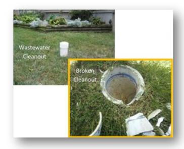
A cleanout is a pipe that appears at ground level and connects to your underground wastewater line. Cleanouts are typically found near your home and close to the property line. Cleanouts have a removable cap on top that allows for easy access to wastewater lines for maintenance and repairs.
