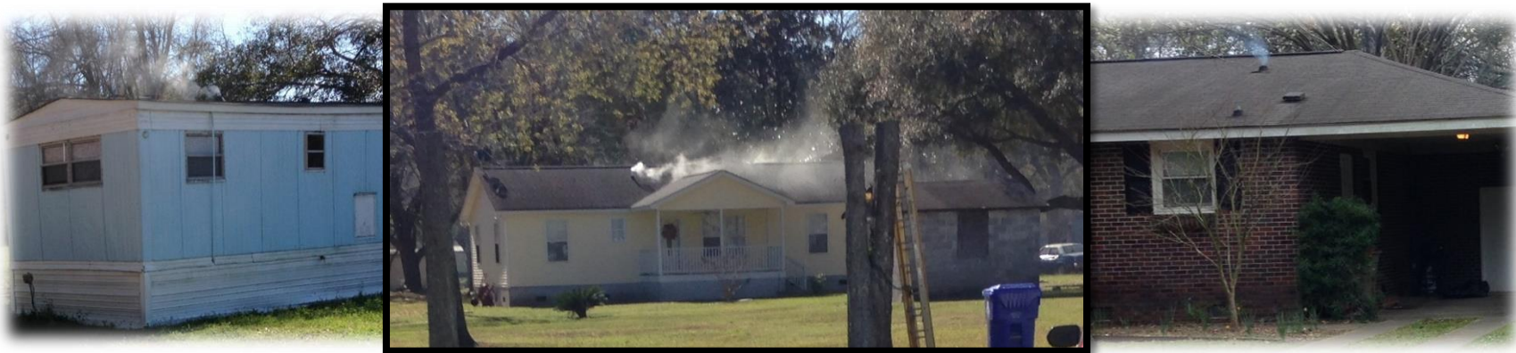
Roof vents properly working during testing
